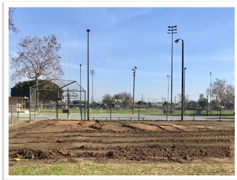
Tee-ball field renovation in progress
